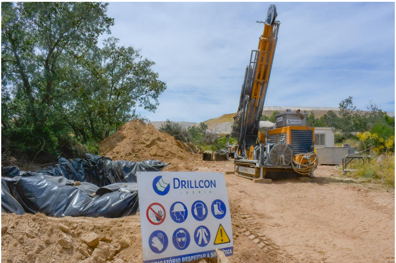
Figure 1: Drill rig on site at Barruecopardo Mine
