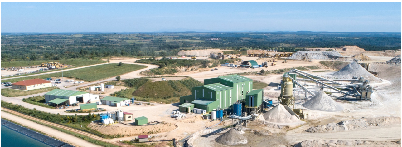
Fig.2 - Barruecopardo Site: Looking from North to South; in front the main processing plant with the crushing & screening circuits to the right
