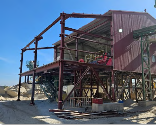
Pictured above left: the existing building containing the two ore sorters being extended to make room for the third ore sorter. Picture above right: the ore sorter distribution hopper installation progressing.
