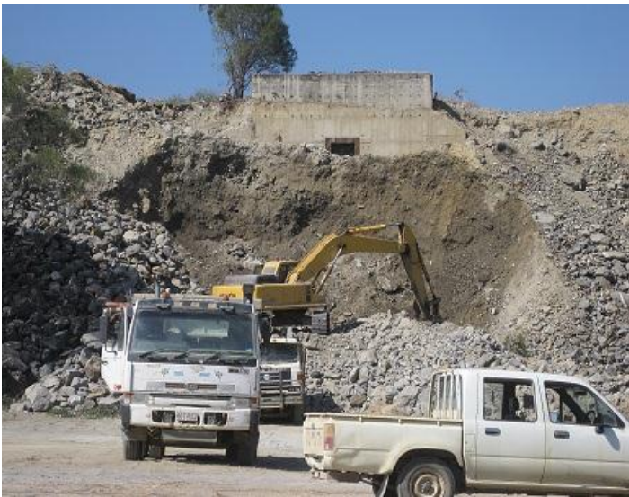
Clearing of existing hard rock crusher civil structures
