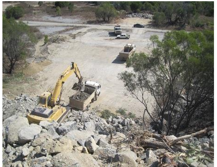
Hard Rock plant pad clearance
