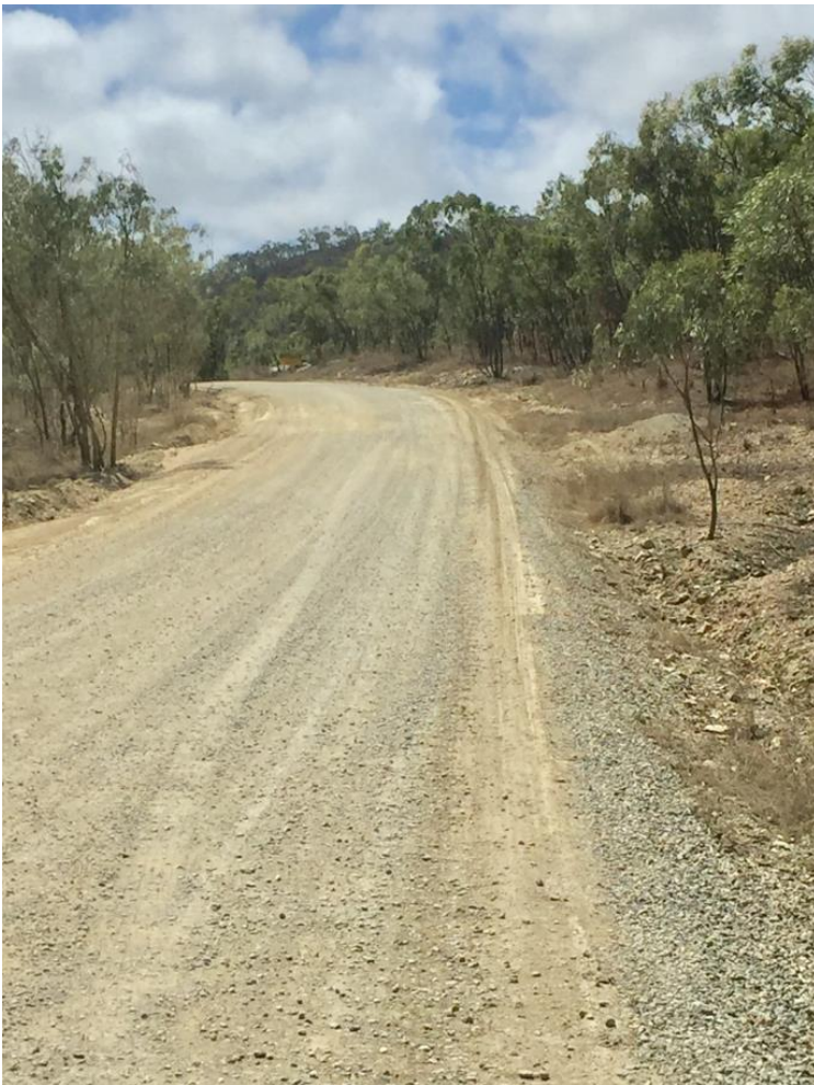
Figure 2: Site Access Road
