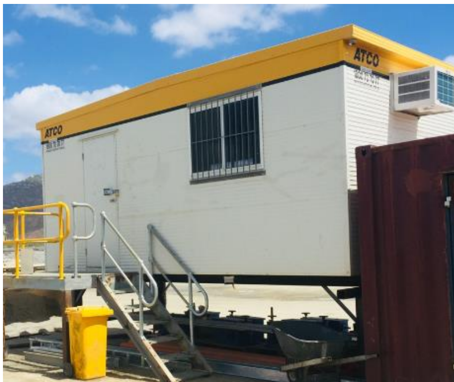
Figure 15: Example Office Building
