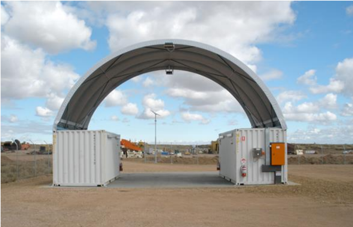
Figure 12: Typical Igloo Workshop
