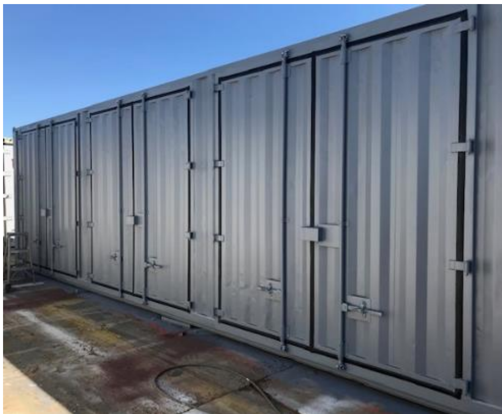
Figure 10: Modified 40ft Container Warehouse
